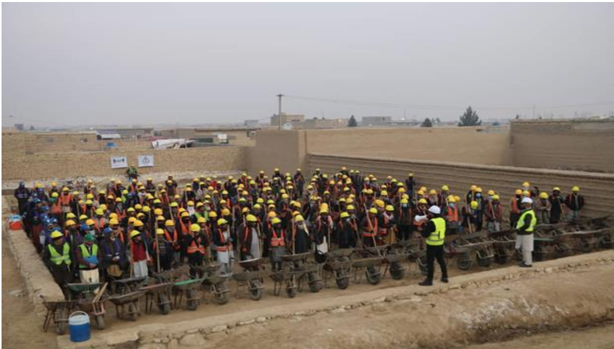
Photo: HSSE induction to the male skilled and unskilled labourers at project site, district#9 of Mazar-e-Sharif
